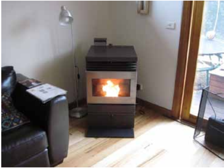
10kWth pellet heater; space heat for house in South Caulfield. Photo David Coote
