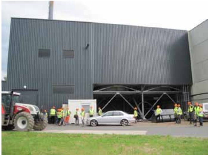
2MWe cogeneration plant in Lower Austria. Photo David Coote
