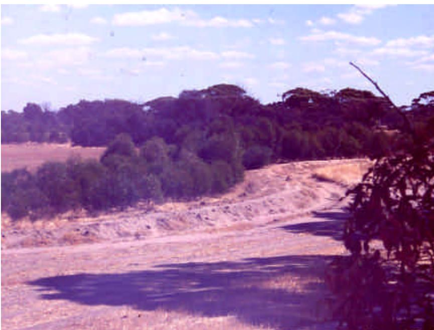
Photo 9. A grade bank which aims to move water to a natural drainage line. Trees are planted behind the bank to maximise utilisation of water that infiltrates the soil.
